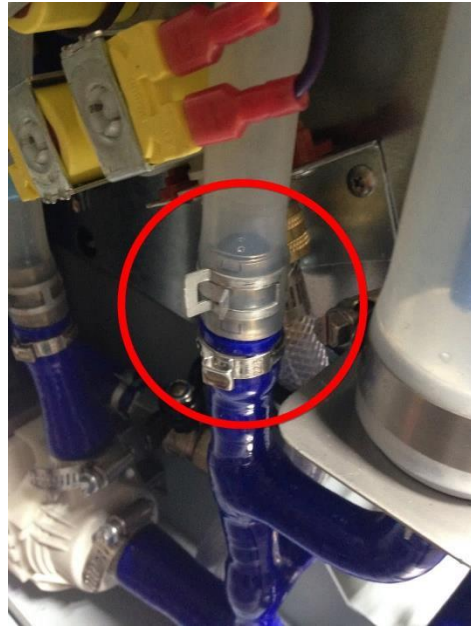
Connect the condensate hose
